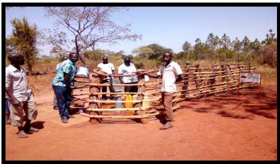
One of the water sources constructed by the project
